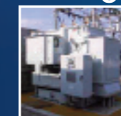
Transformer Drying / Filling
